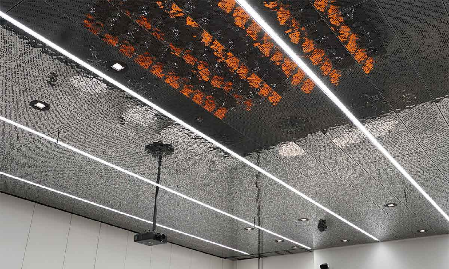
2016 · Sindelfingen, Daimler, Vehicle Safety Technology Center · Architects Heinle, Wischer and Partner · Ceiling System LINDNER, Ceiling Panels EXYD-M · Photo EXYD
